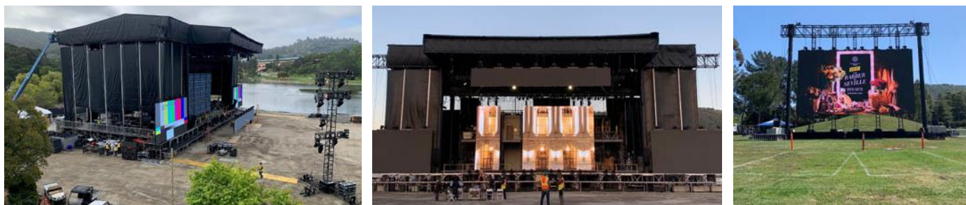
Construction of SF Opera stage at the Fairgrounds, Marin Center; Tech rehearsal showing projection; Simulcast screen at the Lagoon, Marin Center
